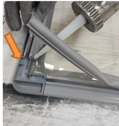
*Fig 16.c. Insert the new seal in the seat of the lid profile.*
